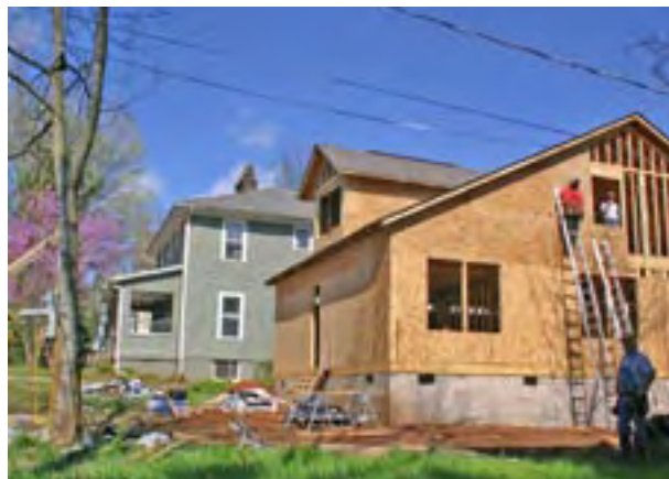
Work continues on infill housing in Old North Knoxville.
