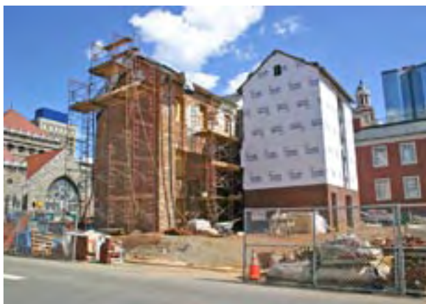
The Park House in downtown Knoxville is being restored.
