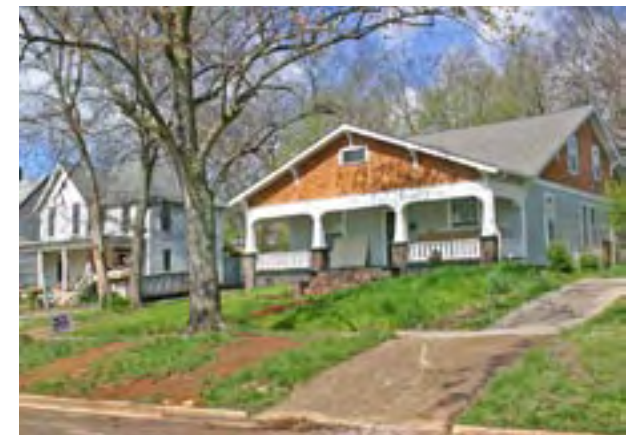
Two homes on Oklahoma Avenue are rehabilitated.
