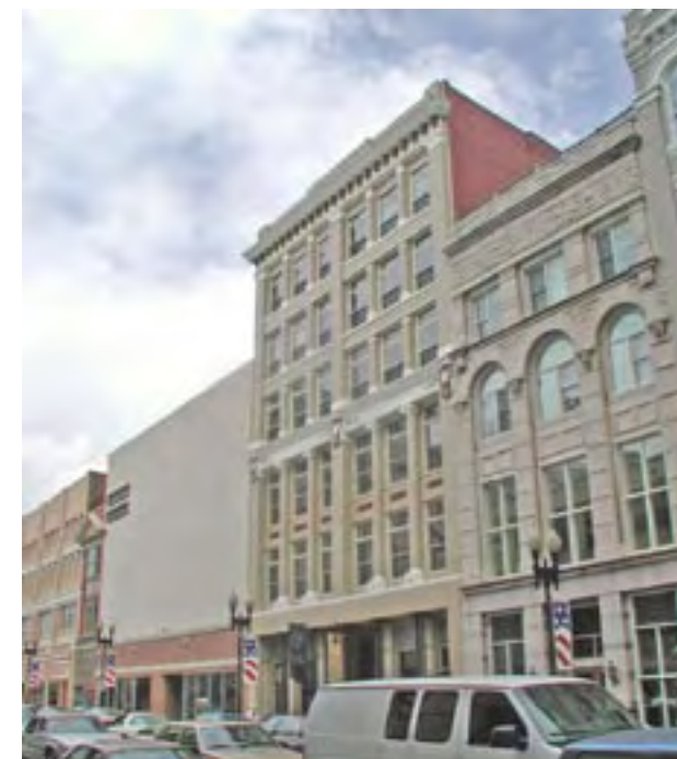
The restored Phoenix Building on Gay Street utilizes the mixed-use philosophy, having loft apartments on the upper floors, office space in the middle and a variety of retailers on the ground level.
