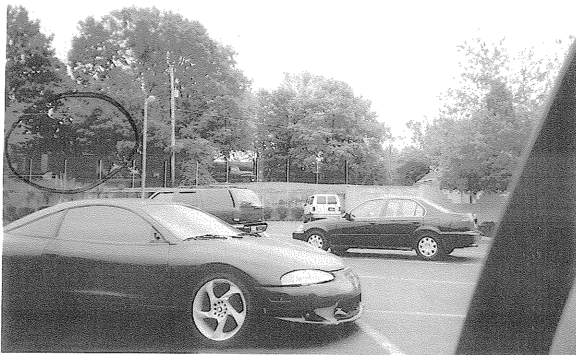
PICTURE OF RETAINING WALL AT THE BACK PARKING AREA WITH THE PATIO LOCATED AT THE RIGHT OF THE PICTURE. THIS PICTURE ALSO SHOWS THE CLOSE PROXIMITY OF NEIGHBORING HOUSES
