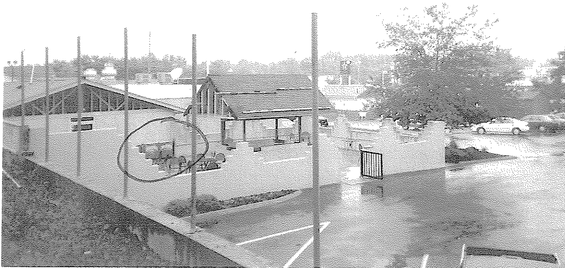
ICEHOUSE BEER COOLERS AT THE ENTERANCE TO THE PATIO AREA ALONG WITH VIEW OF RETAINING WALL AND FENCE POSTS ALONG RETAINING WALL
