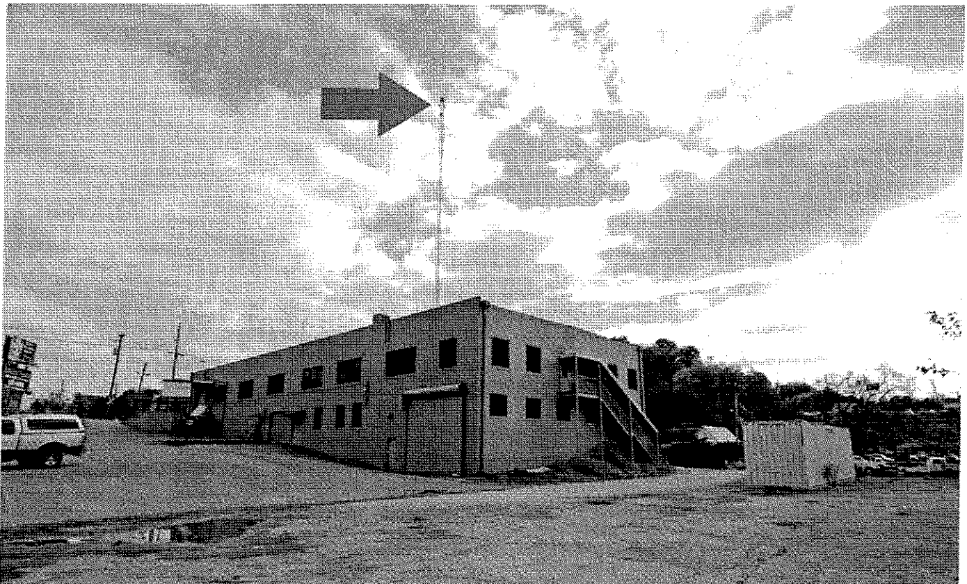
Existing 125 foot tower
