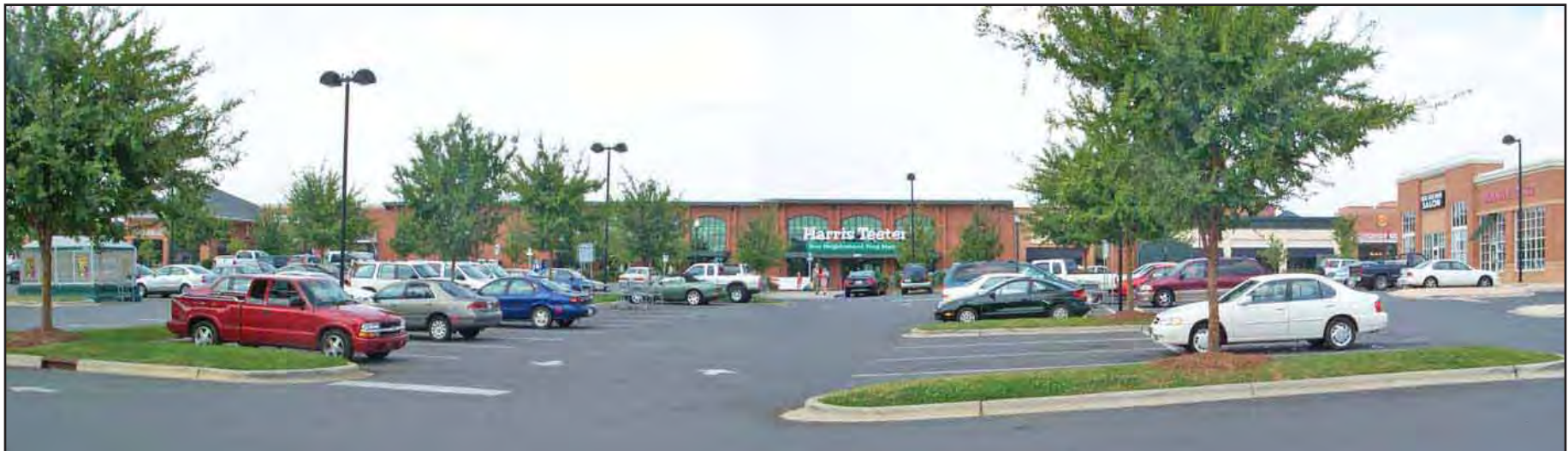
Bottom: One tree per 10 parking spaces is recommended for shade and visual relief.
