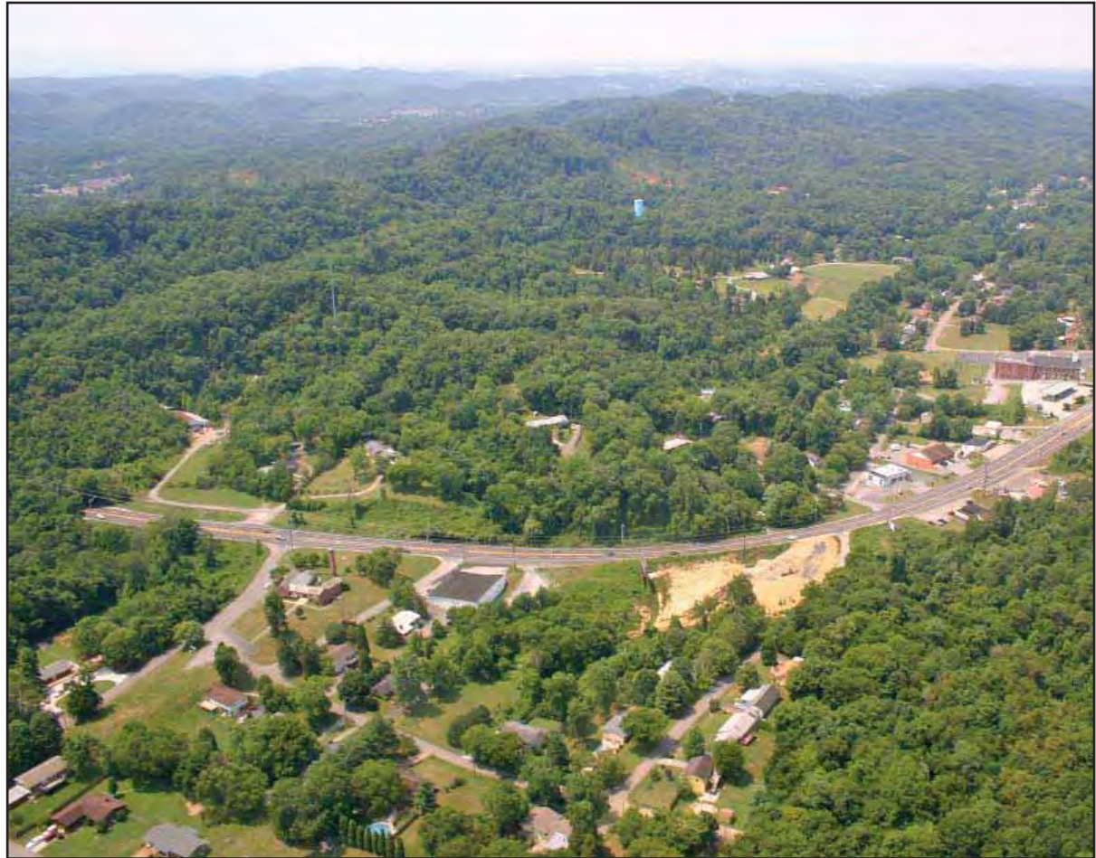
The portion of Chapman just south of Ellis Road near E. Dick Ford Lane has no center turn lane or median. The James White Parkway-Chapman Highway Corridor Study Task Force, meeting in 2004-2005, recommended to TDOT that the James White Parkway extension not intersect with Chapman Highway in this location.
