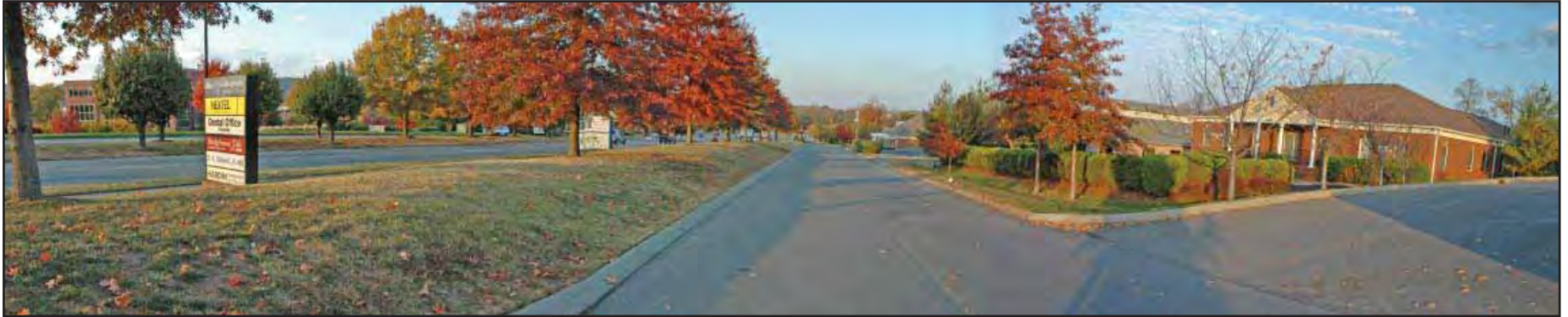
A frontage road is used to provide access to businesses along this corridor. Monument signs and sidewalks are located in the street yard adjacent to the main arterial.
