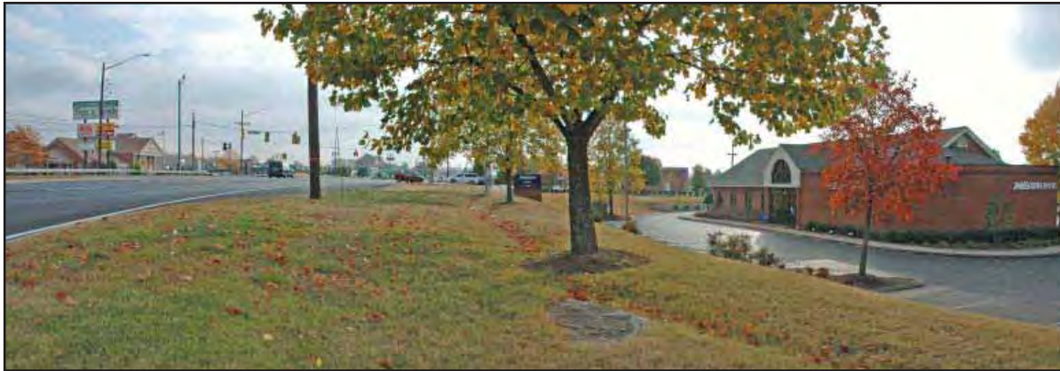
This suburban building is enhanced by quality materials, a monument sign and landscaping that softens the parking area.
