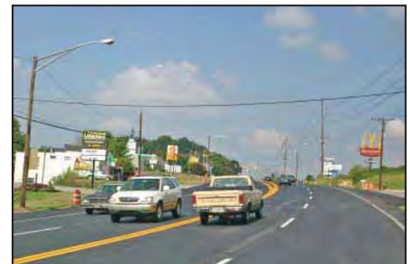
Sections of Chapman have no center turn lane or median.
