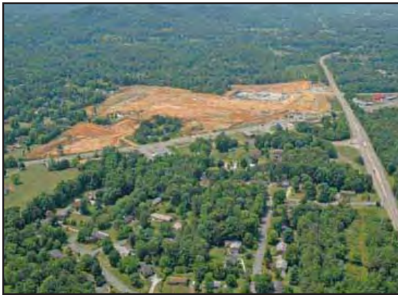
Site preparation is under way on the Southgrove development.
