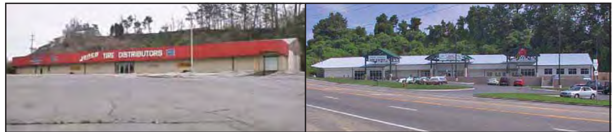
SOUTH TRADER'S LANDING: The metamorphosis of a decrepit tire warehouse into an attractive shopping center. The wall signs provide information about the tenants without relying on large pole signs, and landscaping softens the parking area.
