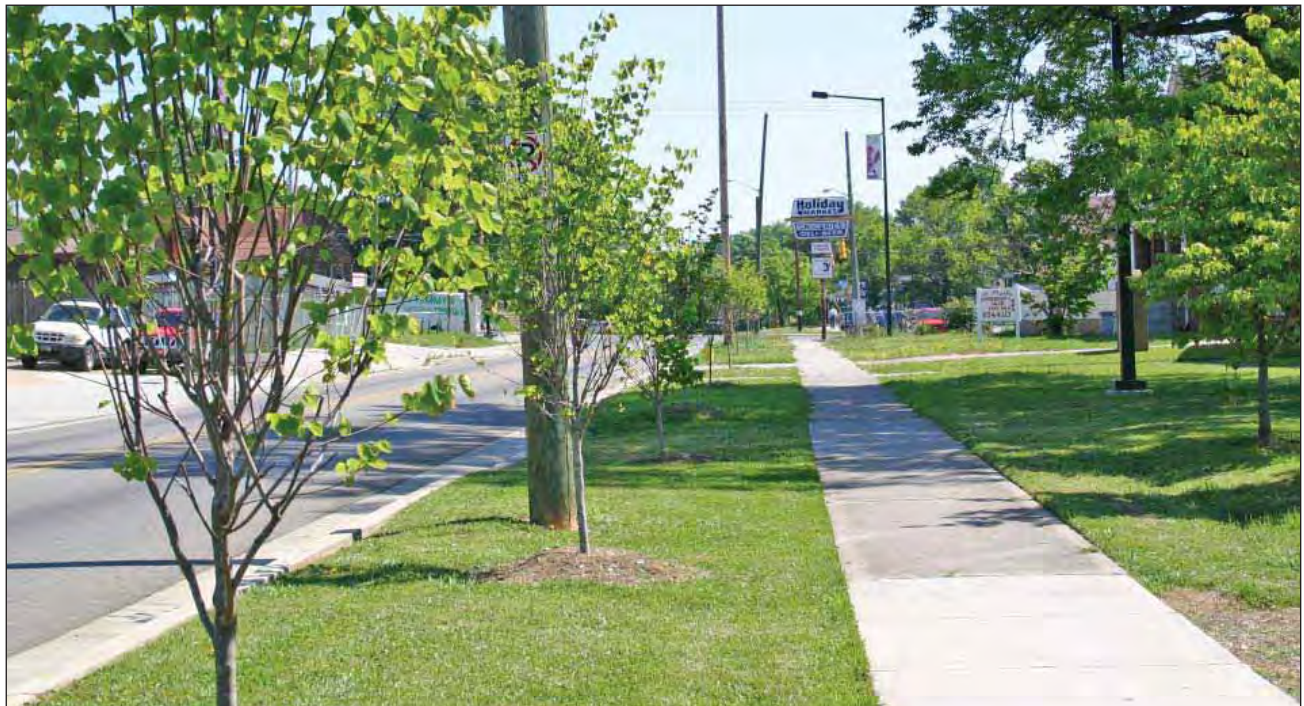
The south side of MLK, Jr. Avenue has been redesigned to make walking safe and pleasant.
