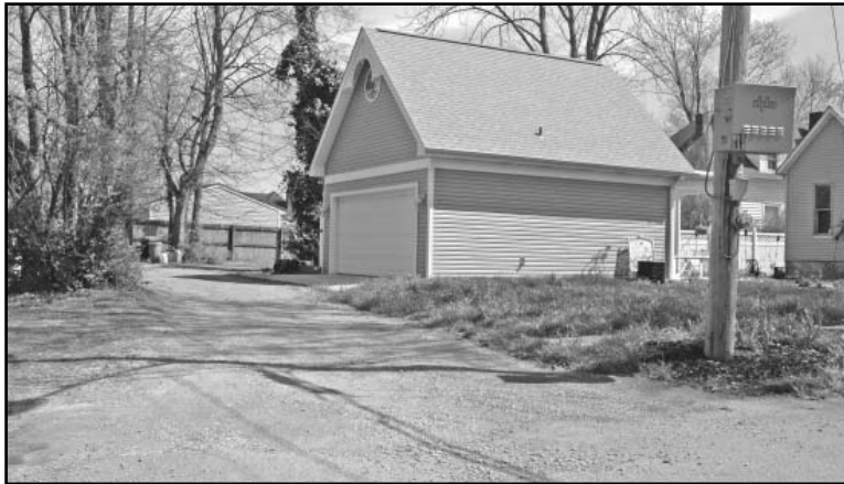
A new garage located off an alley on Oakwood Avenue.
