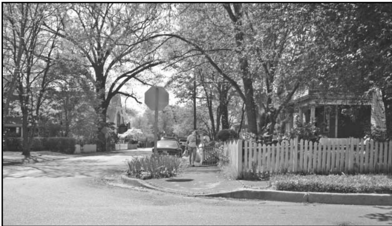
Example of a "bulb-out" at the end of a block in the Fourth and Gill neighborhood.
