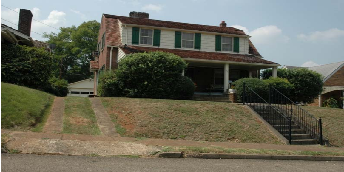
Garages and off-street parking should be located behind houses. Eight-foot-wide driveways or concrete strip driveways (see above) are allowed.
