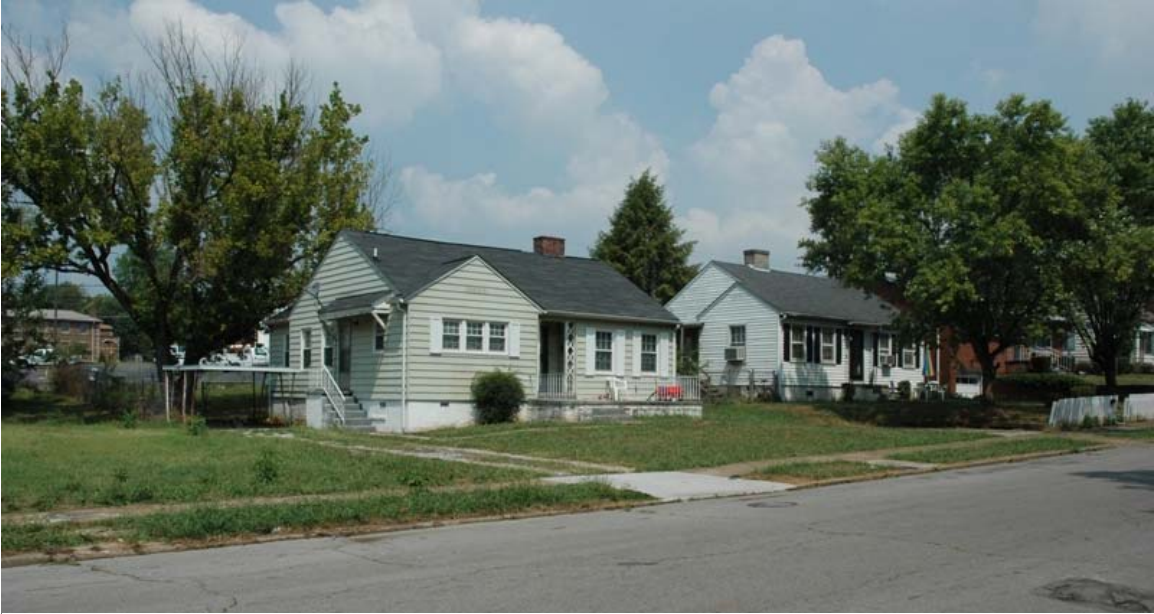
Porches and roof changes (to allow a steeper pitch and additional upstairs space) can be permitted on ranch-style houses.
