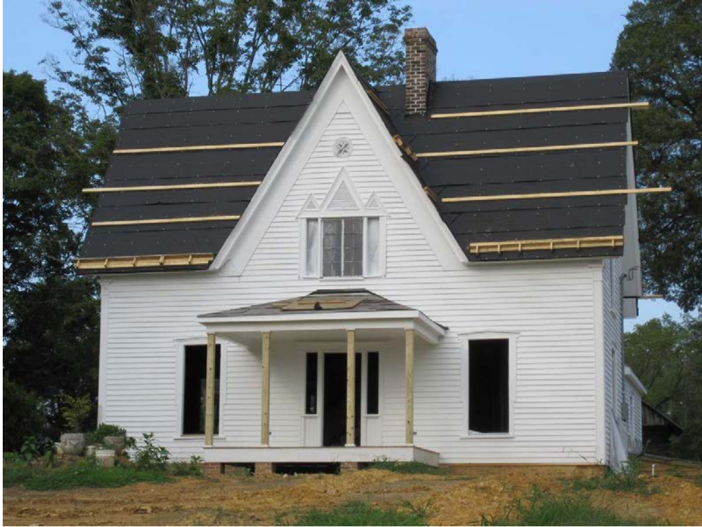
Figure 12 – Recent picture of the ongoing restoration of the Hugh Murphy House
