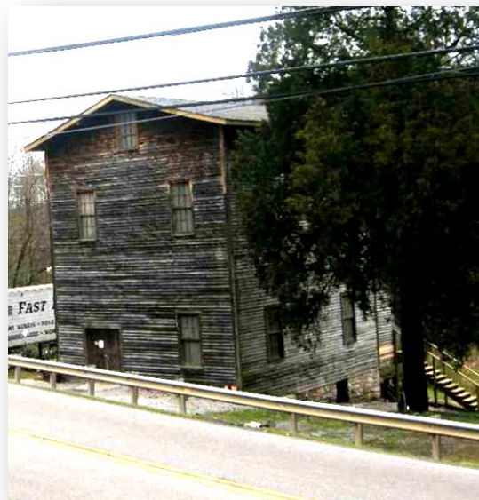
Charles McClung was given a permit to run Ebenezer's Mill, on S. Ebenezer Road, in 1797. The original structure owned by town planner McClung burned, and this mill was rebuilt around 1870 at the same site. It is on the National Register of Historic Places and is one of the very few places in the county to have H-1 zoning.
