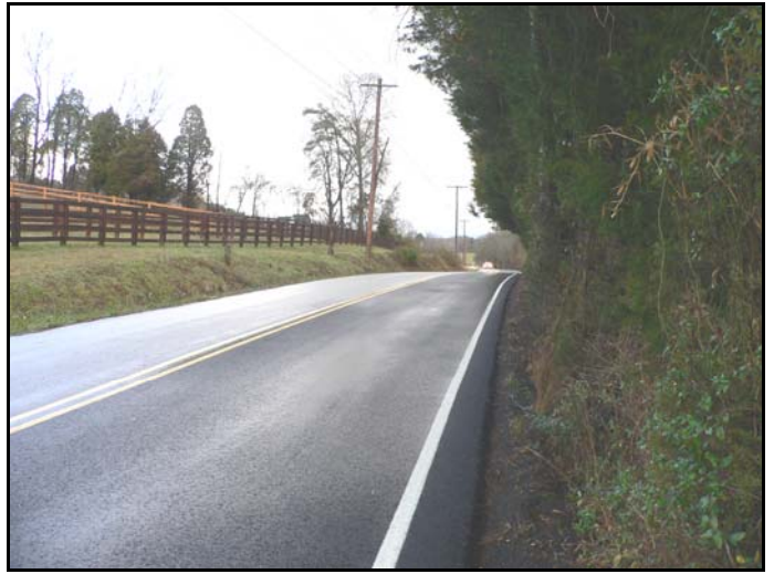
View of Hickory Creek Road from Proposed Roadway Tie-In (Looking Northeast)
