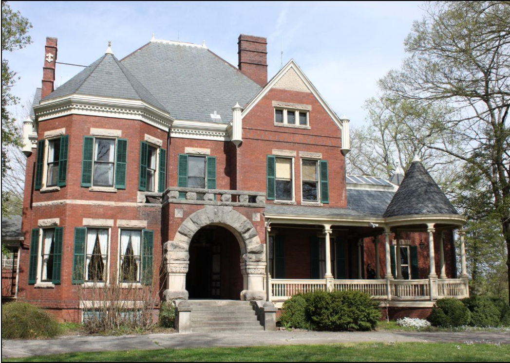
Westwood – Facade.south elevation
