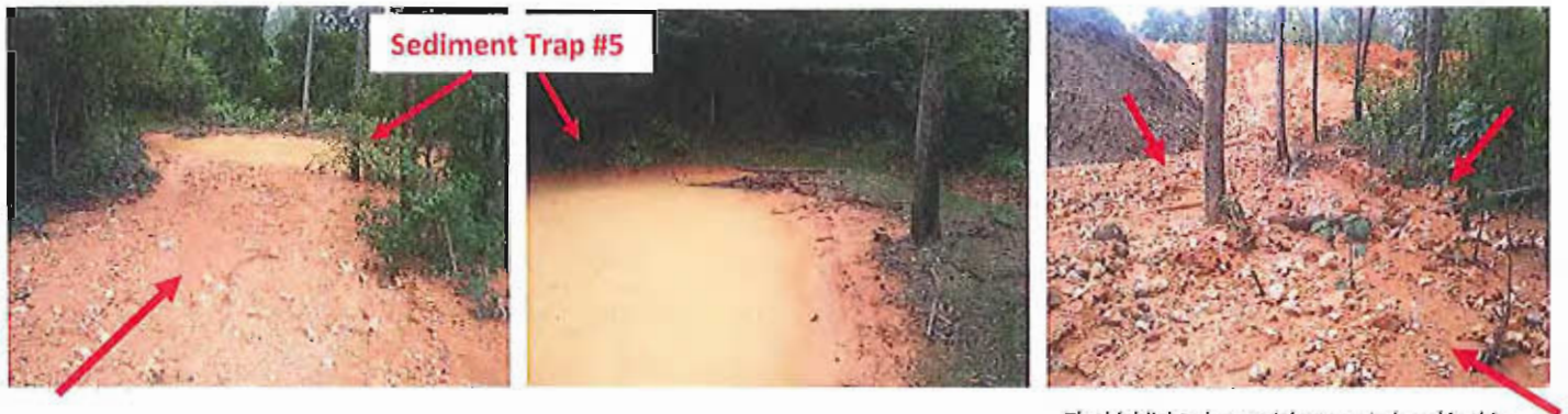
This sediment has washed into the sinkhole and must be removed.
