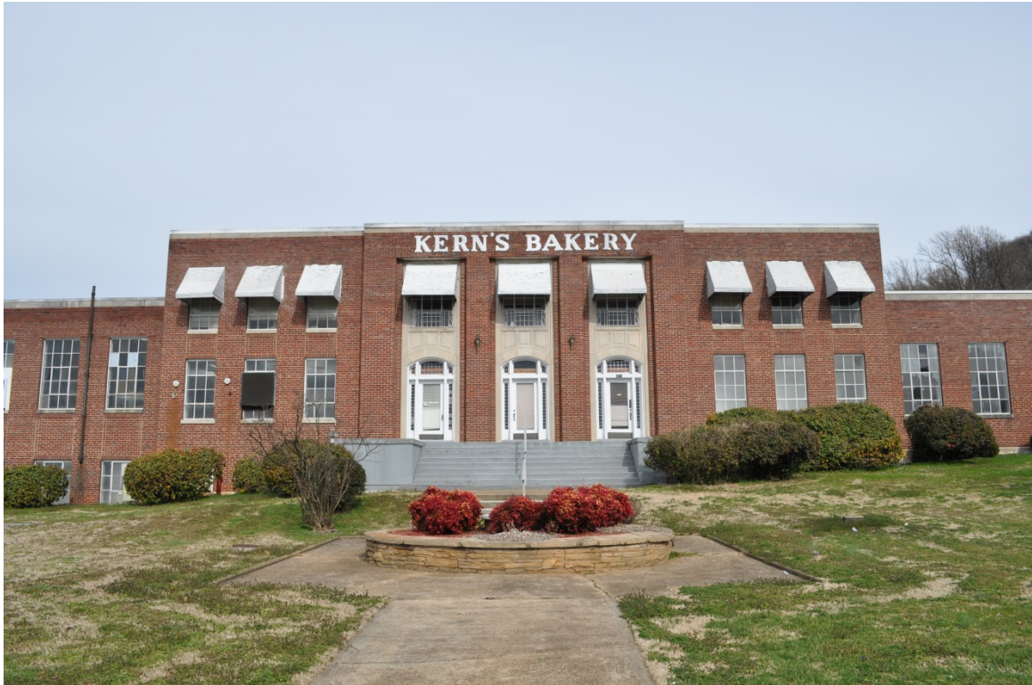
Kerns Bakery – Front façade, center section
