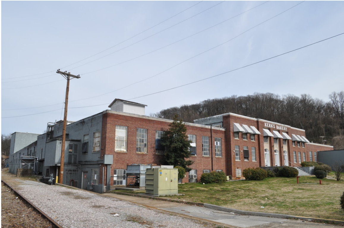
Kerns Bakery – North facade
