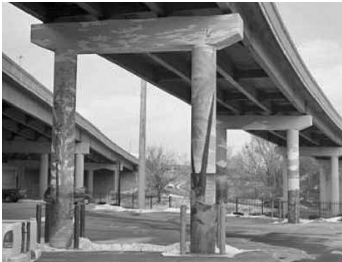
Painting is an inexpensive way to improve underpasses
