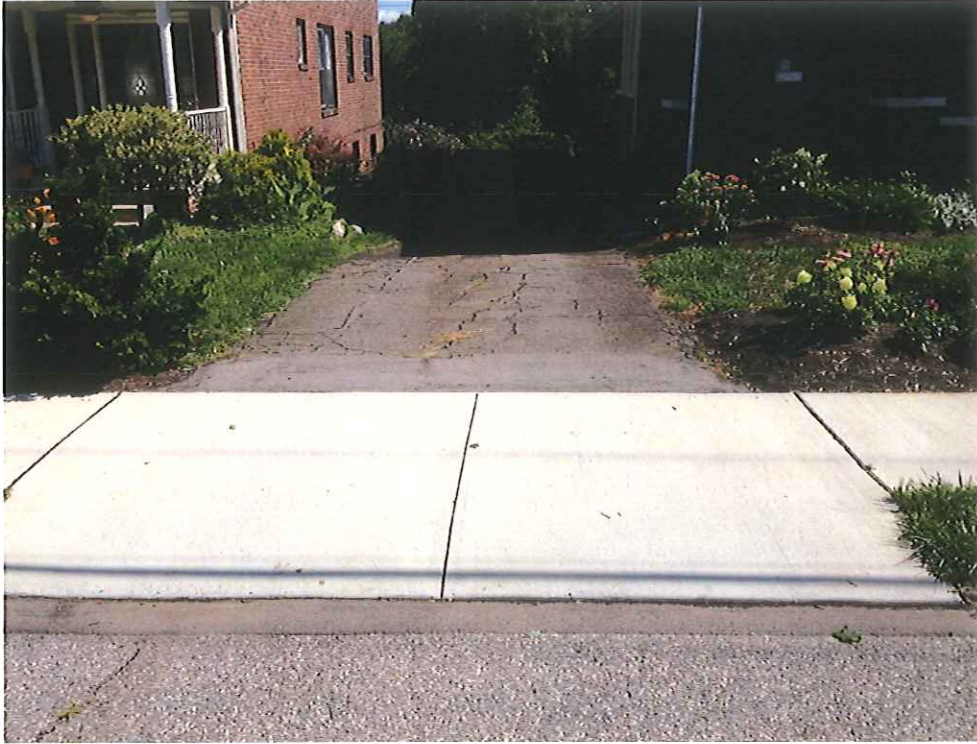
Driveway at curb.
