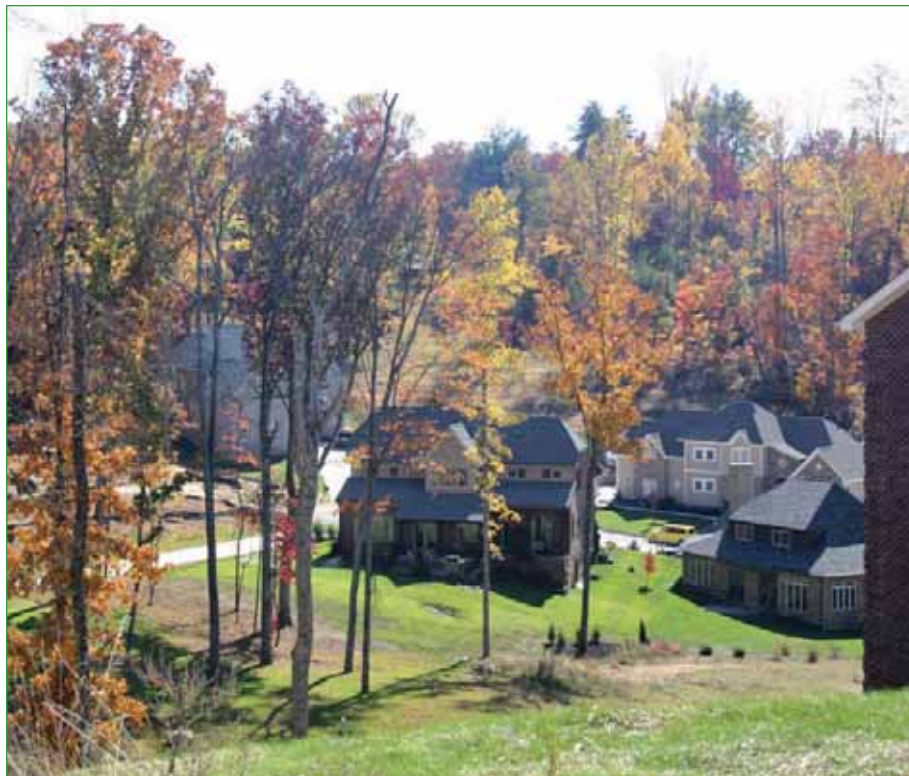
An example of two dwelling units per acre in the 15 to 25 percent slope group
