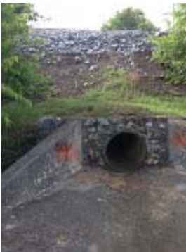
Drain pipe on proposed development.JPG 552K
