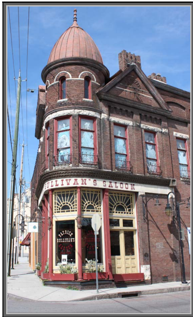
Patrick Sullivan's Saloon prior to current renovation.
