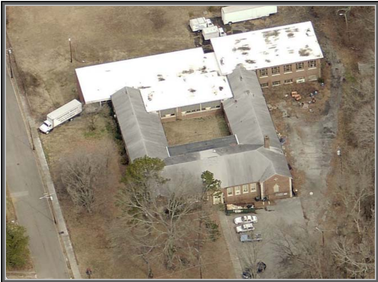
Bird's-eye view of the former Giffin School building.
