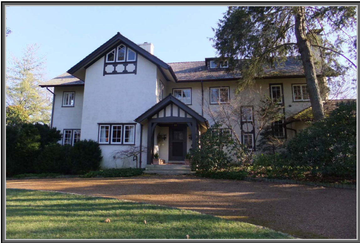
Front façade view of the 1915 Hilltop House showing Craftsman detailing.
