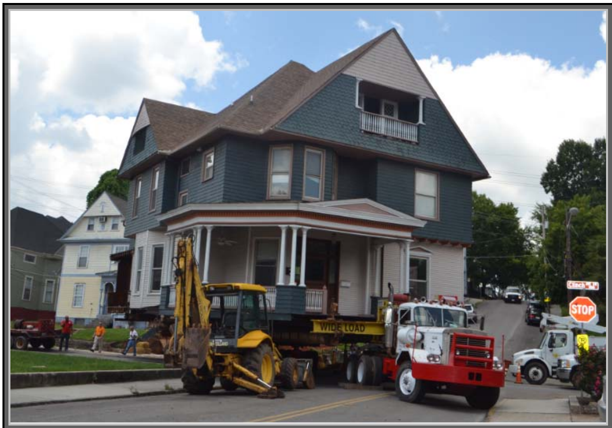
1302 White Avenue was relocated to 1201 Clinch Avenue in Fort Sanders NC-1 Overlay District.
