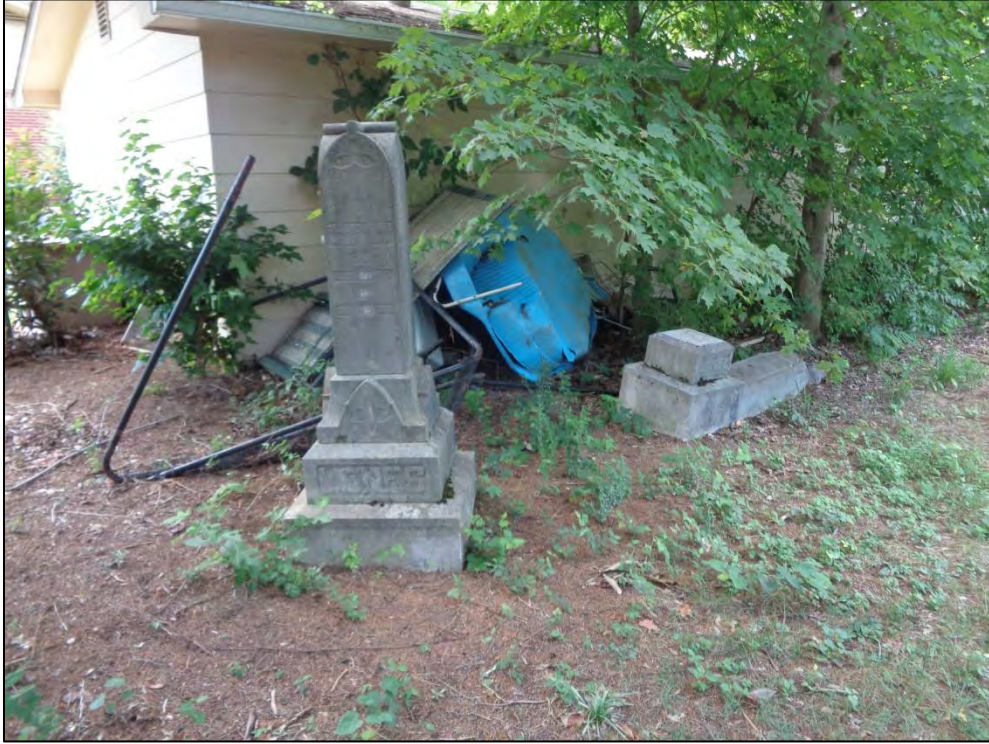
Figure 10. Extant shed and damaged grave marker on the western edge of the cemetery, facing northwest.
