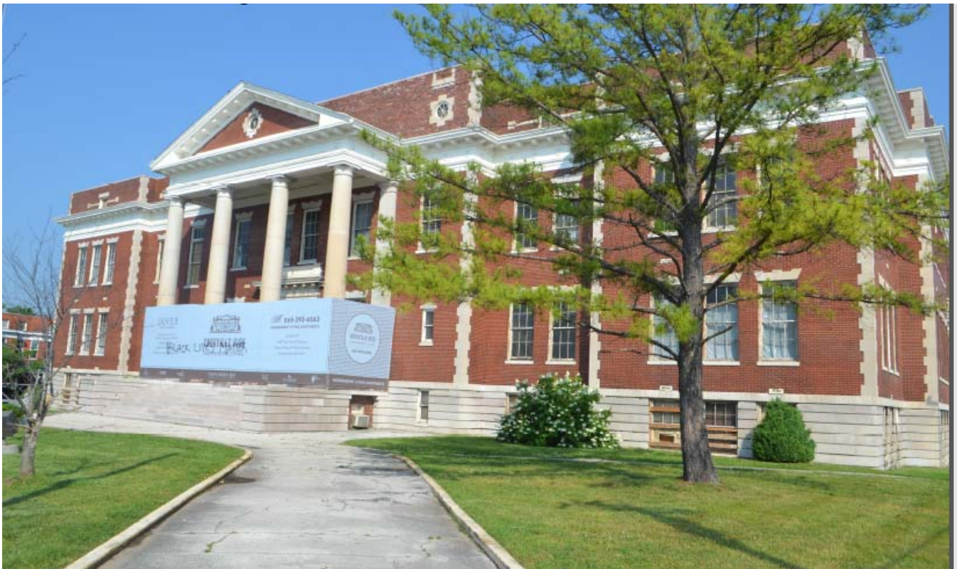
Historic Knoxville High School 2016 – pre-renovation
