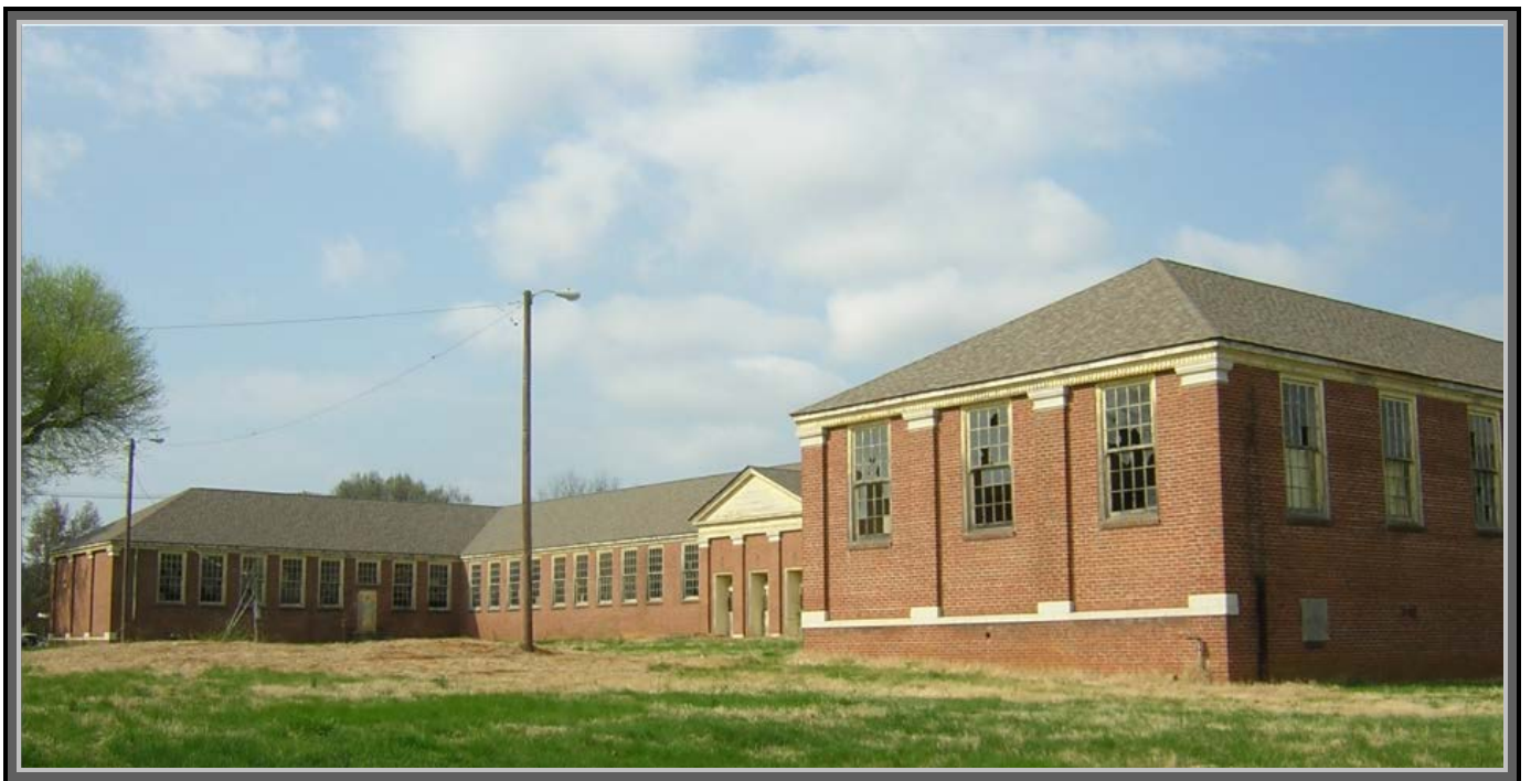
Proposals for re-use of South High as residential units were solicited by the City in 2016.
