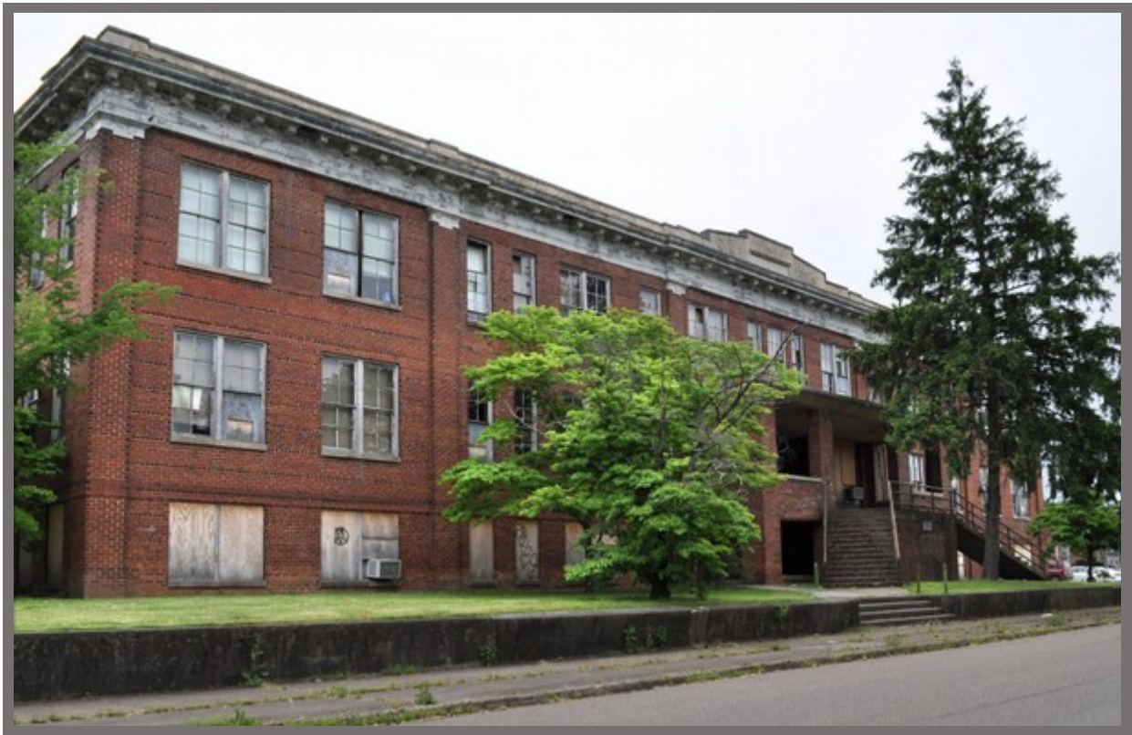
Historic Knoxville High School 2016 – pre-renovation
