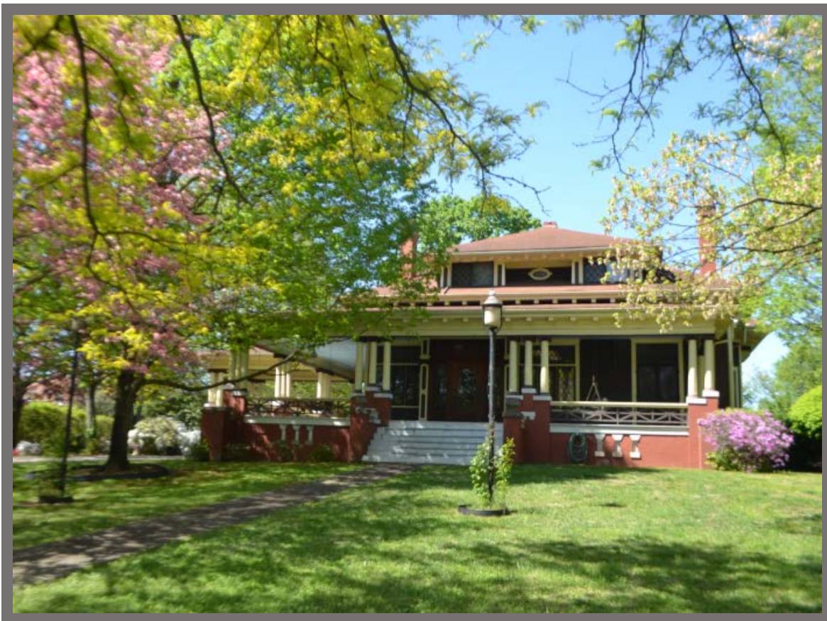
The Howard House as seen from the northeast approach of the circular driveway.
