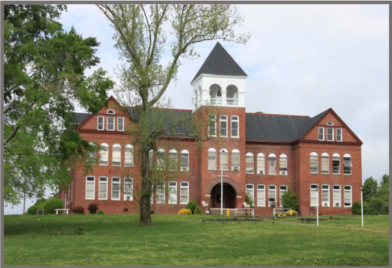
The roof and supporting wall on the rear of the 1876 McKee Hall Administration Building have collapsed.
