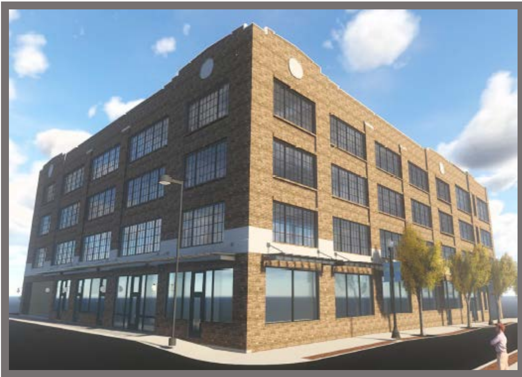
The Pryor-Brown parking garage viewed from the corner of Market St. and Church Ave.
