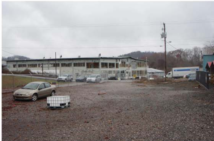
15. View Of Adjacent Building Housing Indoor Field
