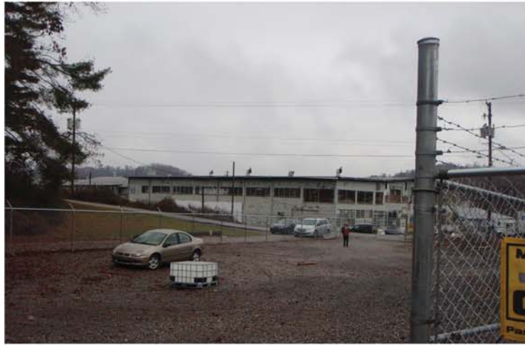
1. Looking Back From Parking To Building With Indoor Field
