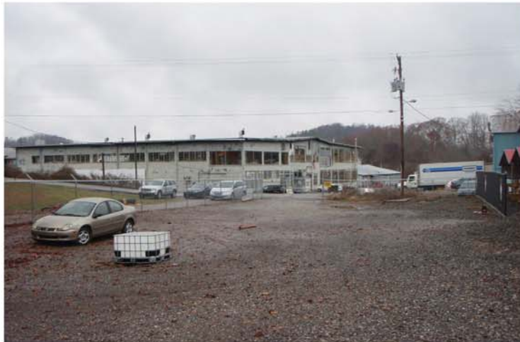
15. View Of Adjacent Building Housing Indoor Field
