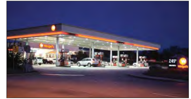
This Weigel's has reduced light pollution impact on adjacent properties.
