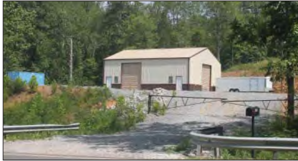
Recently built metal structures in the corridor have spurred concerns by residents over the scenic quality of the corridor.
