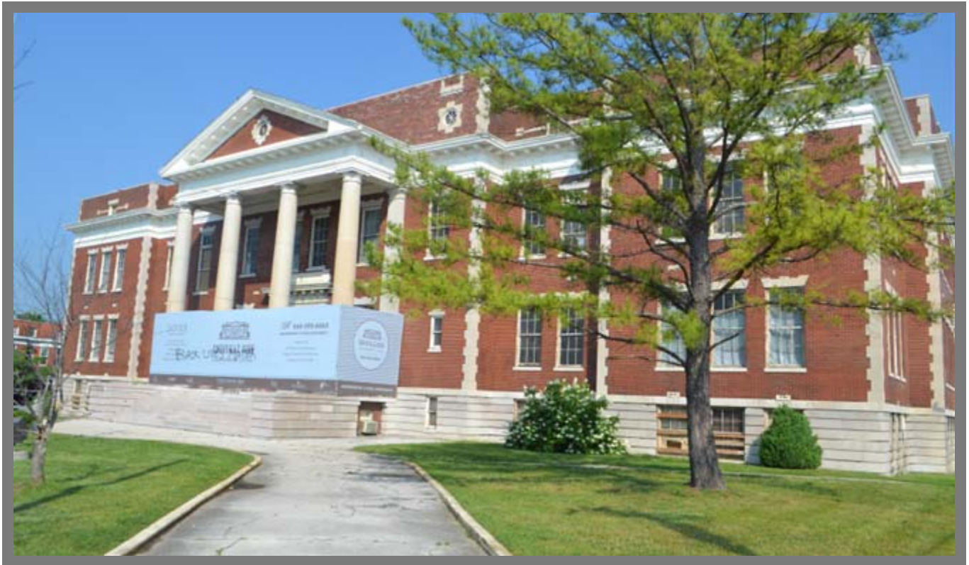
Historic Knoxville High School 2016 – pre-renovation
