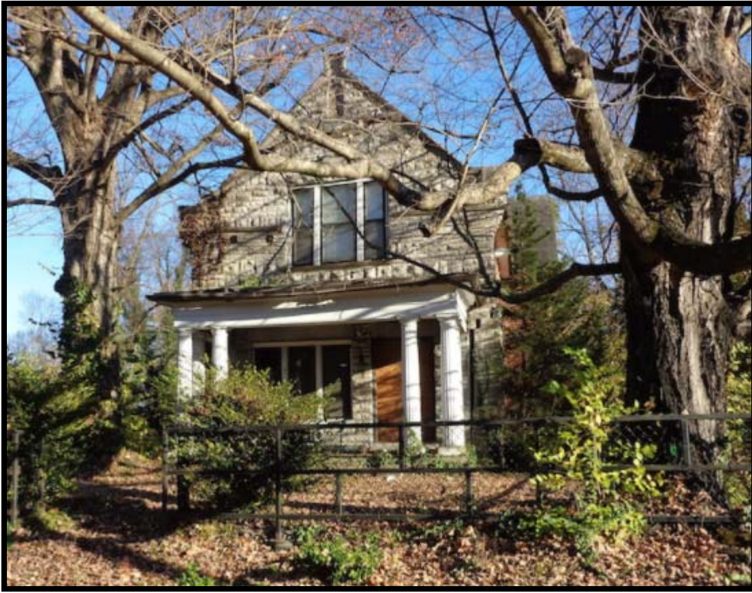
The Knaffl-Stephens House in its later location at 3738 Speedway Circle
