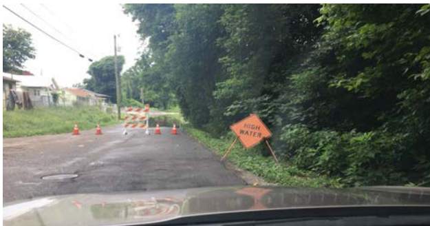
Edington Road on June 28, 2018 flooding did not dissipate for several hours after it has stopped raining.
