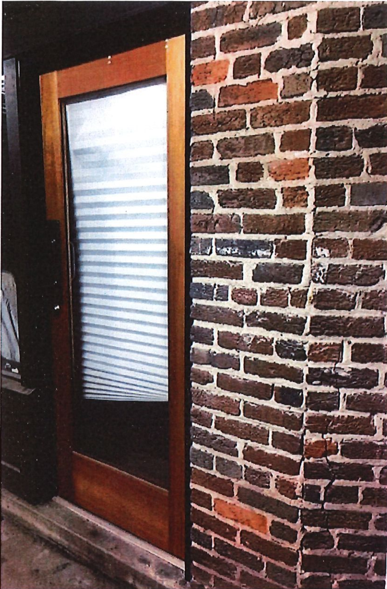
STEEL DOOR, FACING S. GAY STREET, UNDER THE ENTRANCES TO THE FURNITURE STORE AND APARTMENTS WHICH CANNOT BE OPENED FROM OUTSIDE, WHICH LEADS TO COMMON AREA WHERE BACK DOOR OF DSP CAN BE ACCESSED
