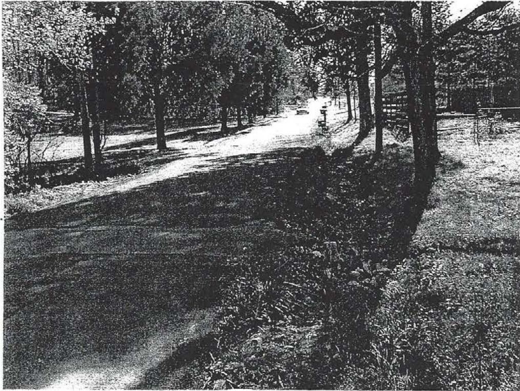
Exhibit 5 Beverly Place looking west from Cloverdale Lane (note: runoff in ditch needs to make 90-degree turn to pass under road through culvert)
