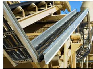
Cable trays on each component neatly keep power and control cables off the ground.
