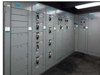
The Astec power house is a secure, climate-controlled, dust free environment.
