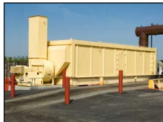
A fiberbed filter unit captures emissions before they escape into the atmosphere.
