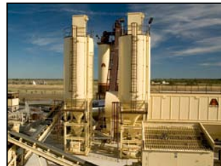
Optional additive silos are used to hold a variety of mix additives.
