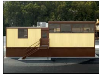
The Astec Command style control house has an elevated control room.
