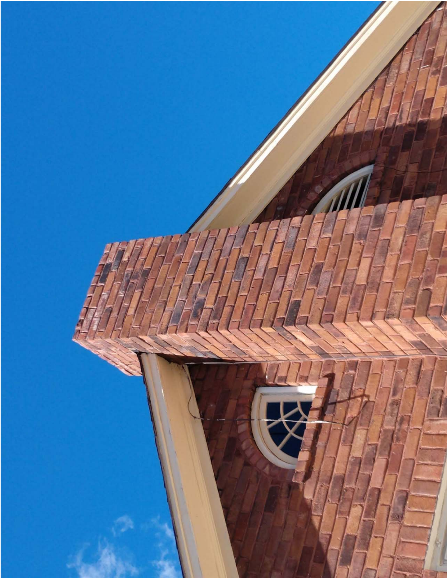
509 18th St. - Chimney and quarter round windows
