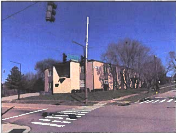
Overall View facing Northeast from E. Fifth Ave. / Winona St. Intersection
