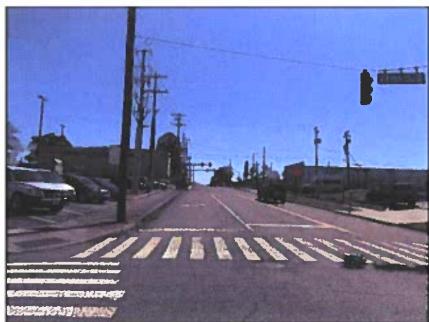
Street Scene – South along Winona St.
