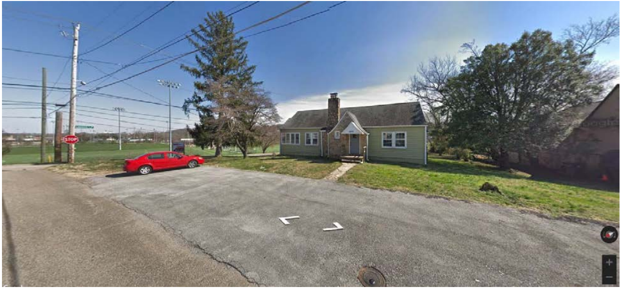
Front of structure facing Chambliss Avenue
