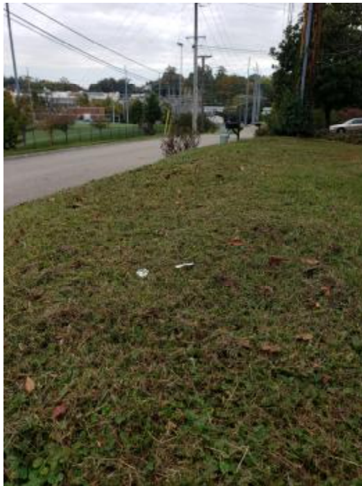
Sight Distance From Ingress/Egress – South
