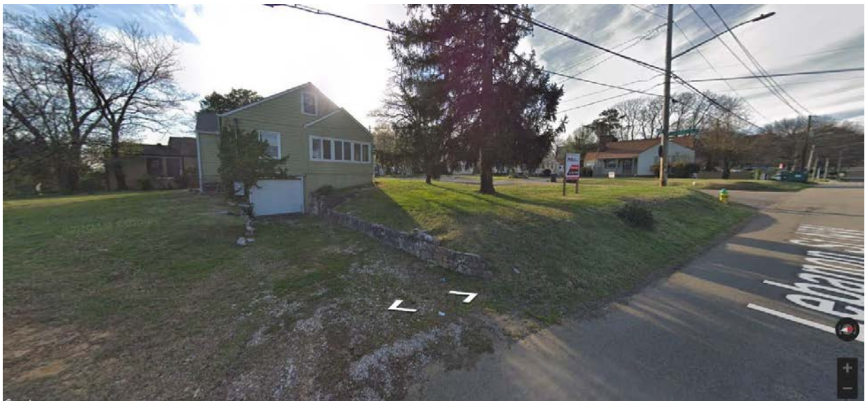
Side of structure facing Lebanon Street
