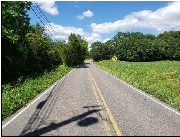
Large trees adjacent to roadway near 420 Brakebill Road with shoulder drop-off into the drainage ditch (Looking North)
