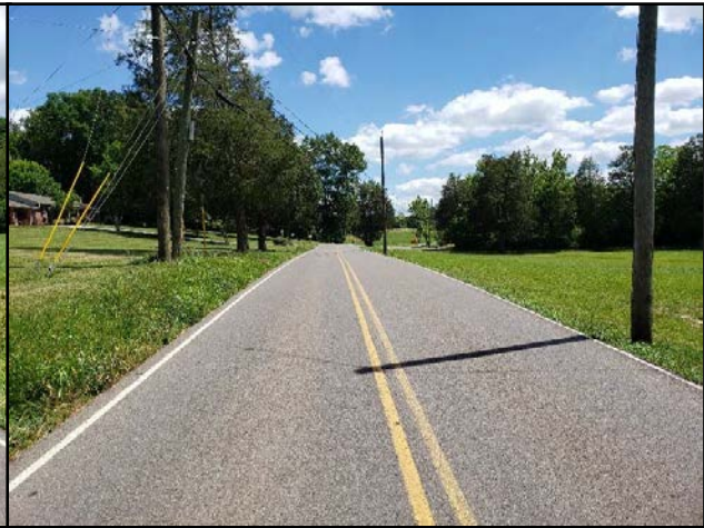
Utility poles adjacent to roadway near 322 Brakebill Road with shoulder drop-off (Looking South)
