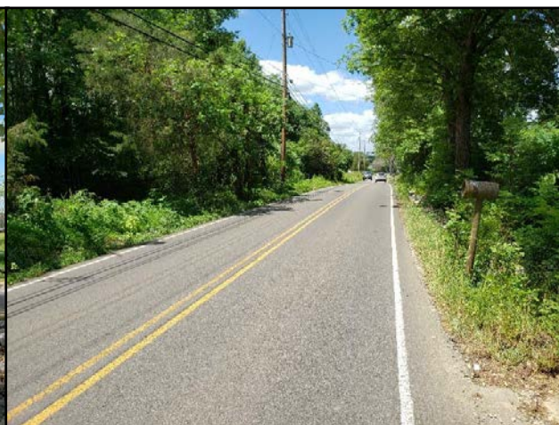
Large trees and utility poles adjacent to the roadway near 508 Brakebill Road with shoulder drop-off into the drainage ditch (Looking North)
