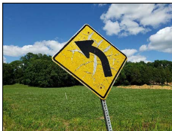
Deteriorated Curve Sign for NB Traffic on Brakebill Road near Kilbridge Drive
