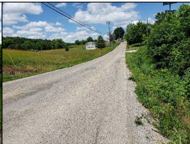
Steep road/shoulder drop-off and deteriorated pavement near 701 Brakebill Road Driveway (Looking North)
