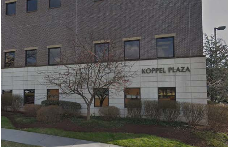
LOCATION 16 SURFACE MOUNTED NON-LIT LETTERING
