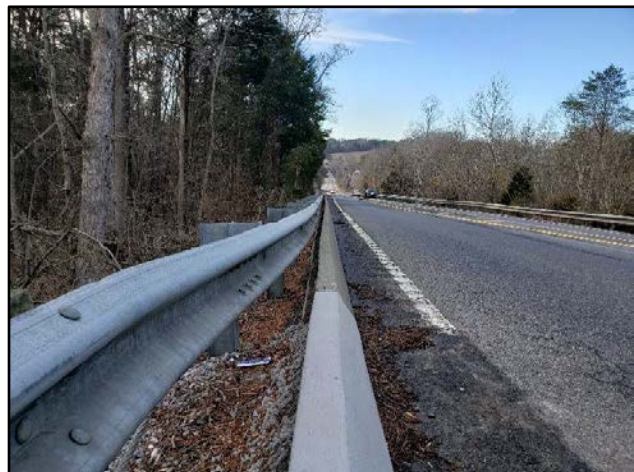
Guardrail and Detached Concrete Curb on South Side of Oak Ridge Highway near Pebblepass Road (Looking West)
