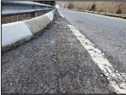
Grooved Rumble Strips on Oak Ridge Highway
