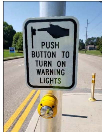
Pedestrian Push Button in Center Median Refuge Area on Ebenezer Road for RRFB
