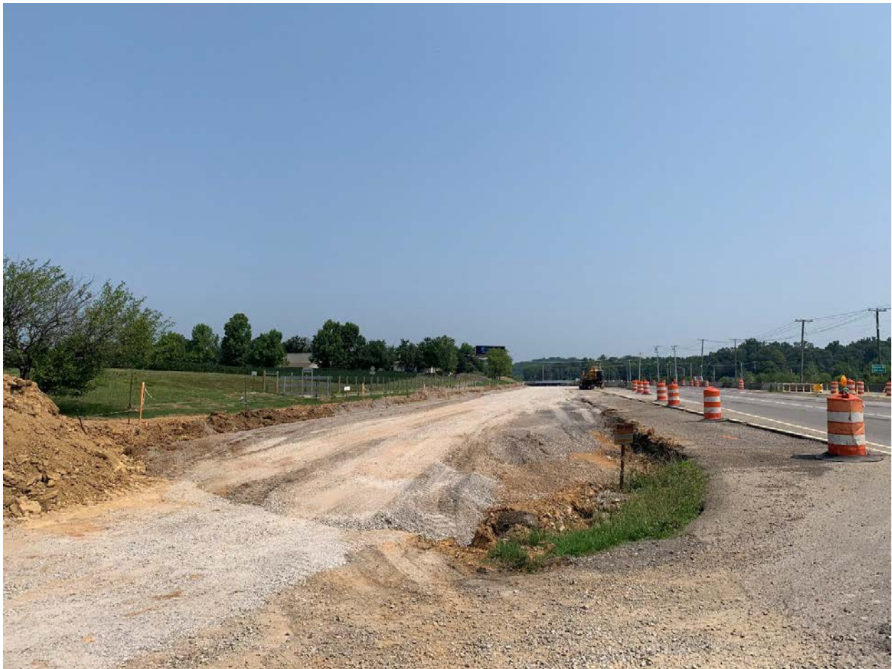
Alcoa Highway construction, July 2021
