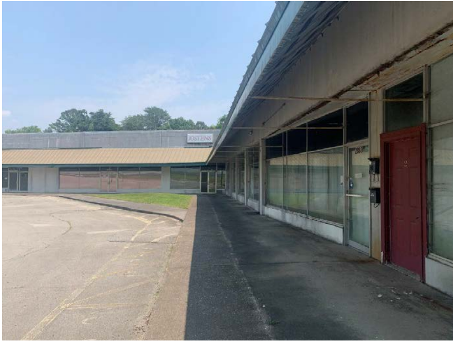
Vacant commercial strip center, July 2021
