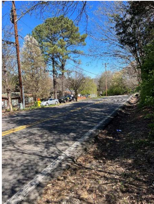
Buffat Mill Road at Roadway Connection (Road "A") – Looking Right
