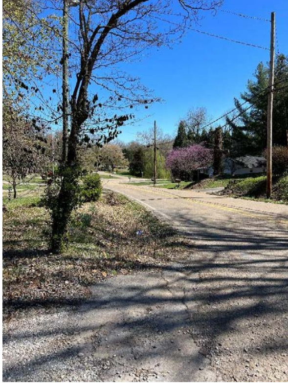
McIntyre Road at Roadway Connection (Road "F") – Looking Left
