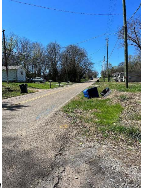
McIntyre Road at Roadway Connection (Road "F") – Looking Right
