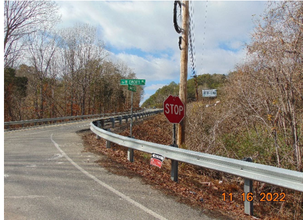
Figure 3: Oak Ridge Highway at W. Emory Rd. ( looking west)
