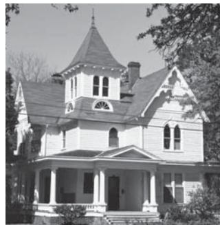
The tower on this Lake Charles Victorian residence is an important part of its design. Were it to be lost, the home’s National Register design integrity would be severely compromised.
