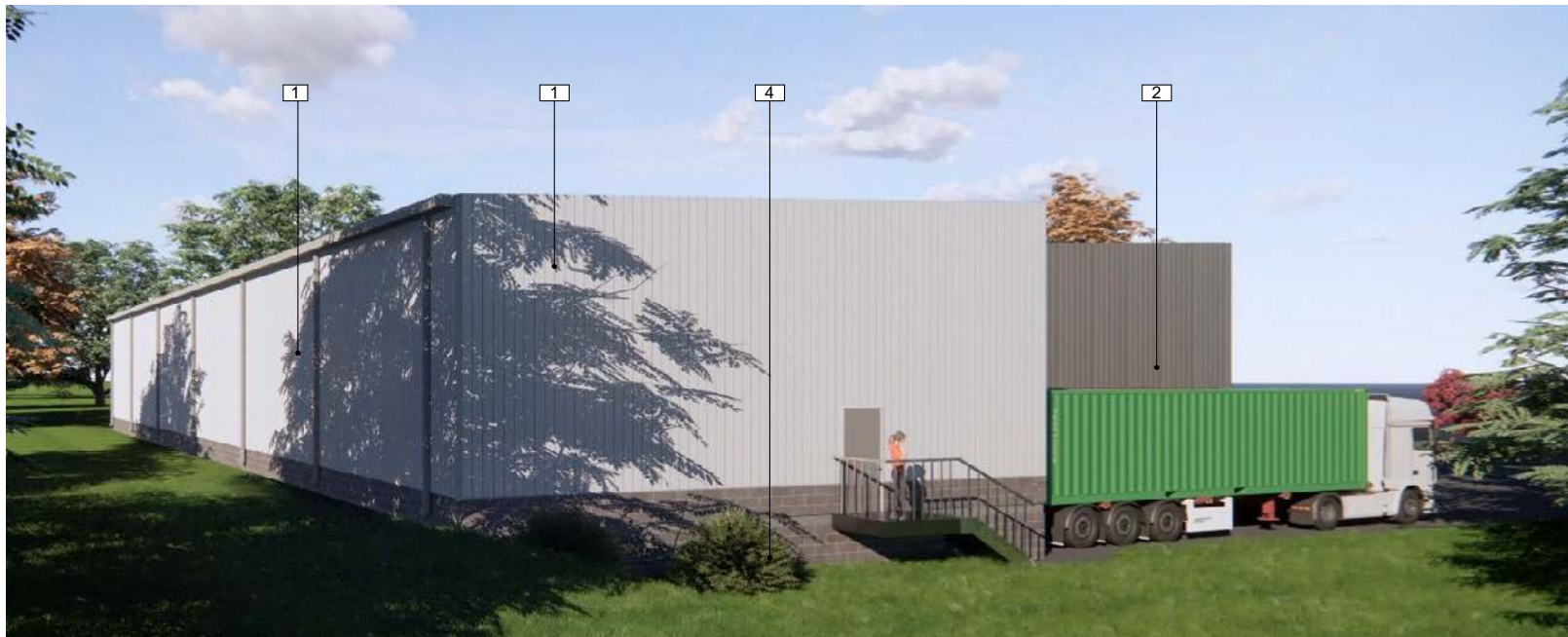
2 SOUTH WESTERN VIEW
