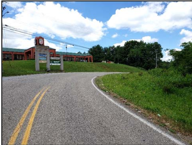
Roadside vegetation obscures sight distance for turning vehicles at Crosswood Boulevard and Brakebill Road (Looking Northwest)
