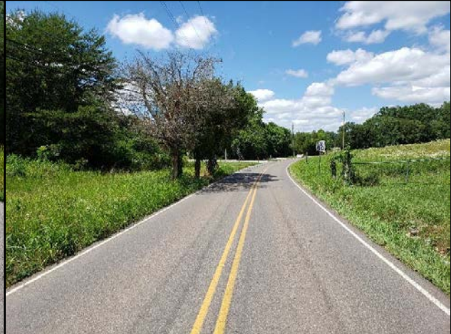
Large trees adjacent to the roadway just south of Kilbridge Drive with shoulder drop-off into the drainage ditch (Looking North)
