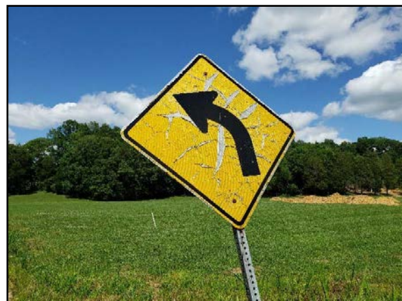
Deteriorated Curve Sign for NB Traffic on Brakebill Road near Kilbridge Drive
