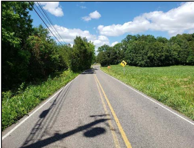
Large trees adjacent to roadway near 420 Brakebill Road with shoulder drop-off into the drainage ditch (Looking North)
