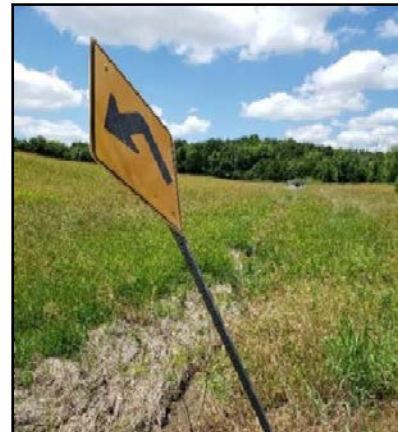
Leaning Sign near 604 Brakebill Road
