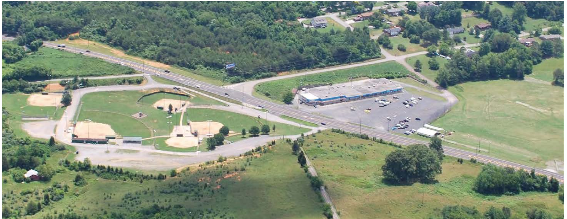
Existing commercial zoning and infrastructure at the Highland View Shopping Center, across from Bower Field, make redevelopment as a mixed use district plausible.
