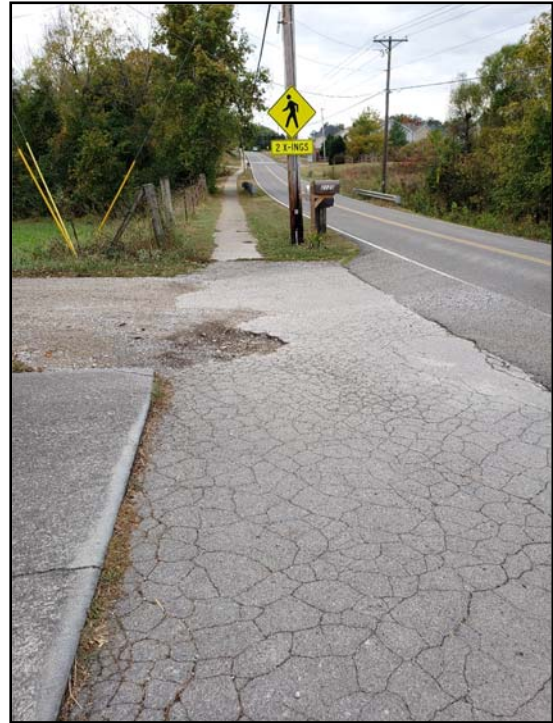
View of Sidewalk Crossing at the Existing Gravel Driveway (Looking West)
