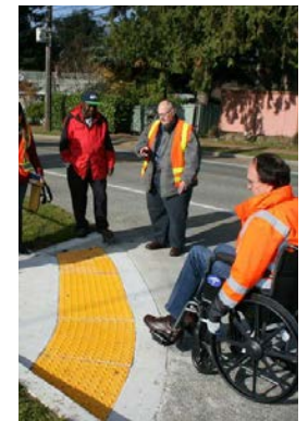
Improvement of existing sidewalks and infrastructure.
