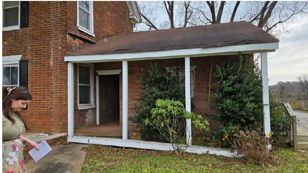
Façade view of 20 th century side wing addition, entrance to side deck
