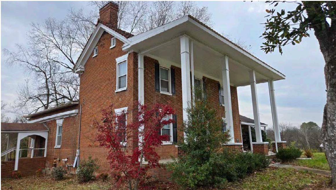
Façade and Left Elevation: original 1805 house, c.1830s rear ell addition, 20 th century front porch
