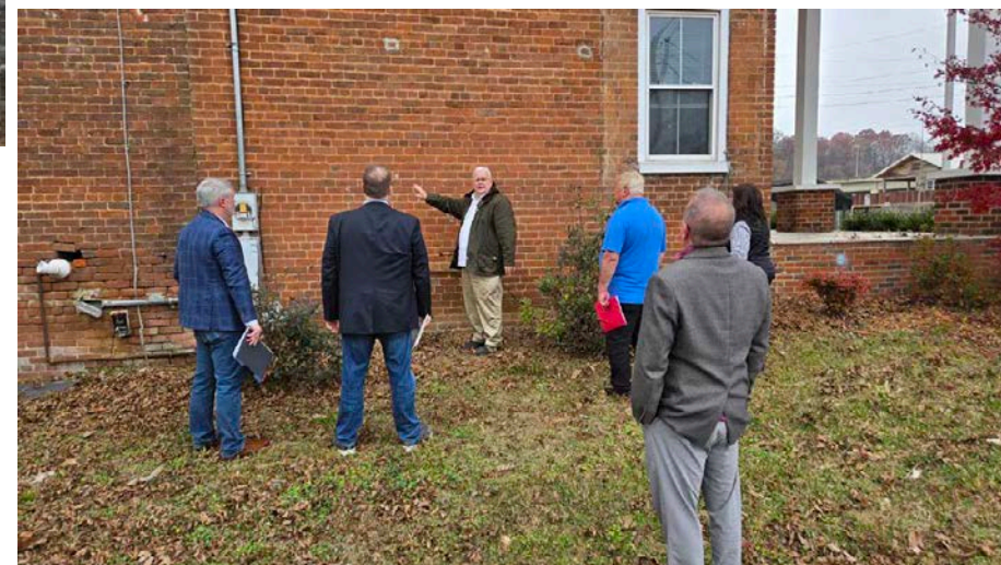
Below: Brick bond differences between rear ell and original house
