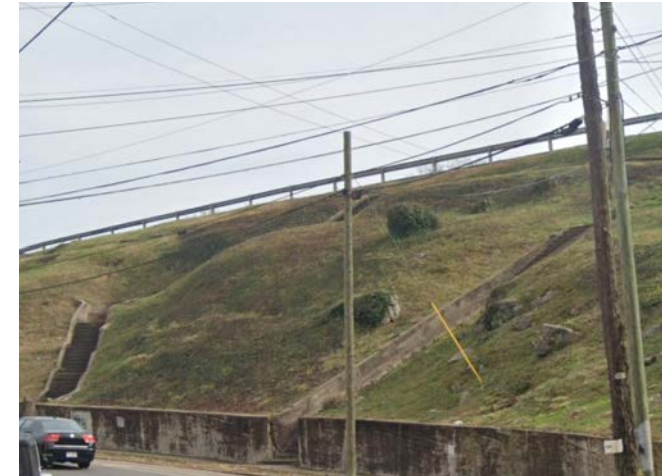
1. Existing Concrete Stairs along Sevier Ave.
