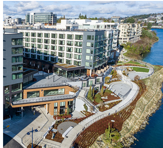
Marina Square Waterfront Apartments | Seattle, WA
