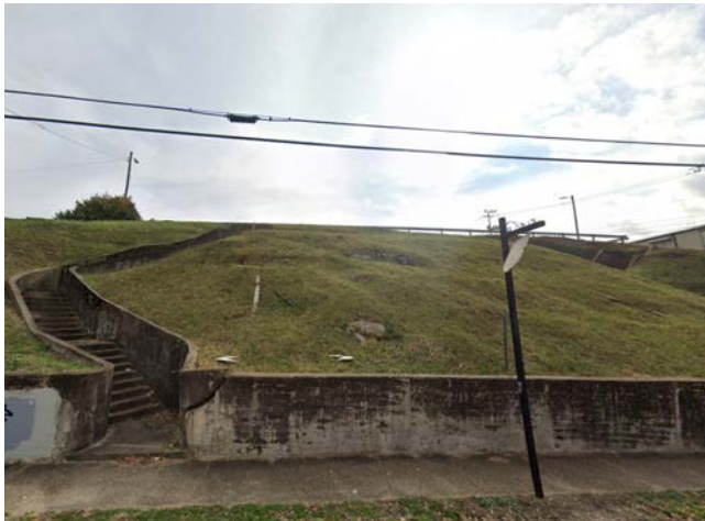
2. Existing Concrete Stairs along Sevier Ave.
