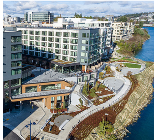
Marina Square Waterfront Apartments | Seattle, WA
