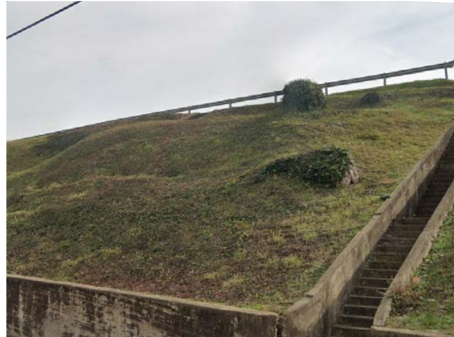
3. Existing Concrete Stairs along Sevier Ave.
