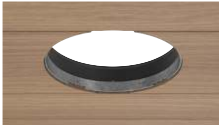
Secure with finishing nails.
